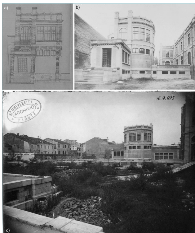
Figure 2. The new “Morgagni Theatre” for dissections: (a) Architectural project from the early twentieth century. (Archives of the University of Padua). (b-c) Photos from 1924/1925 showing the completion of the construction of the “Morgagni Theatre” before the construction of the anatomical buildings. (Archives of the University of Padua)
